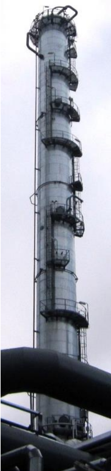
Fig. 1. The rectification column before the accident
